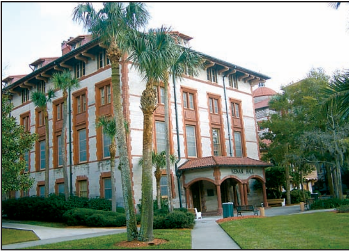
Historic Flagler College enjoyed quiet operation and energy savings after it installed frictionless, magnetic-bearing compressor chillers in two of its buildings.
